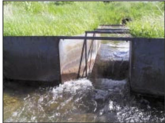
Parshall flumes cause minimal backwater, and work well in low-gradient applications.
