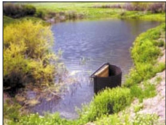
Canal checks, or outflow pipes, are commonly used on small ponds to control water elevations. Canal checks and standpipe structures do not substitute for emergency spillways.
