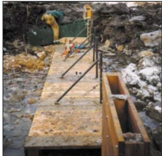
The flat floor and high drop of a pin and plank structure limits fish passage unless fitted with a fish ladder.
