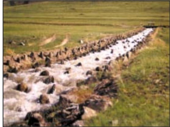
This unique drop structure is a concrete channel studded with rock to slow velocities. Structures are more commonly large rock or formed concrete.
