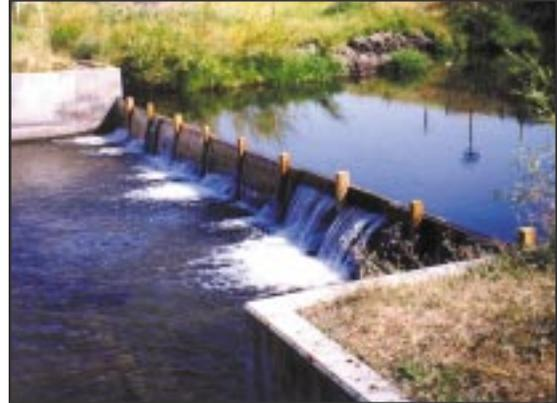
Concrete may be preferred to wood for longevity. This structure is not fish friendly because of the height of the drop and the flat slab downstream.
