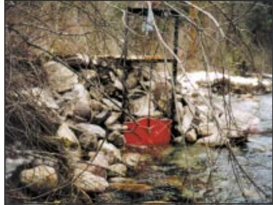
A C-10 gate generally benefits from a headwall to stabilize fill. Rock can work, but the slope leaves the gate frame exposed to ice and debris.
