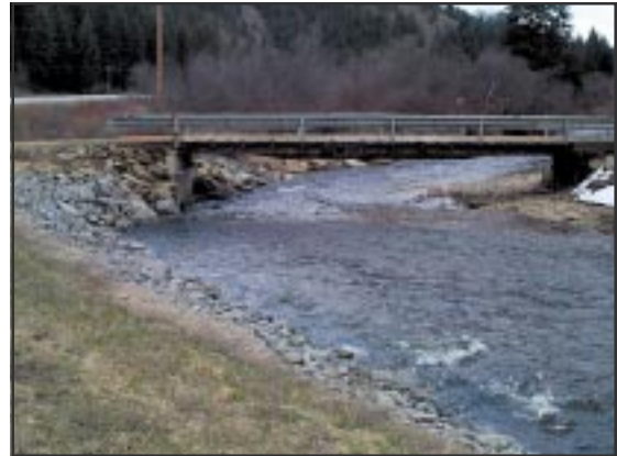
This bridge is set slightly above bankfull, but does not have wingwalls. Location on a meander is not ideal, although upstream rip-rap limits lateral movement. Note that the point bar is still growing under bridge.
