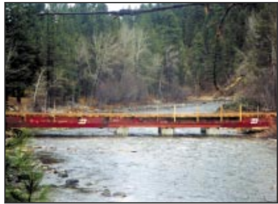
Railcar bridges are popular and fairly solid, but often are not installed properly. This one is set low relative to bankfull, but it is a temporary installation.
