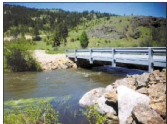
The structural beam on many railcars hangs low and ends up falling below bankfull elevation.
