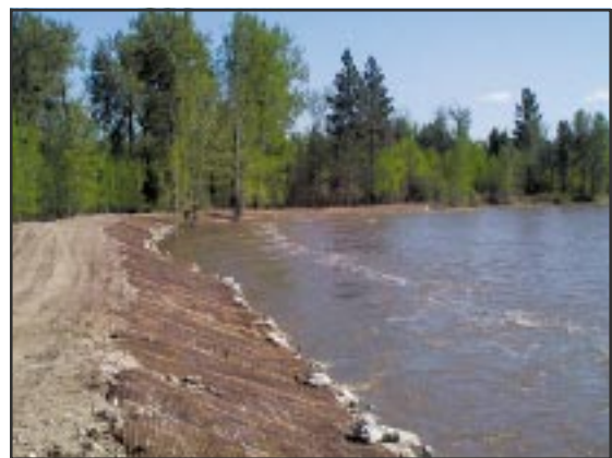
Levees provide flood control for development in floodplains. Levees require ongoing maintenance, however, and have the potential to severely impair channel function.
