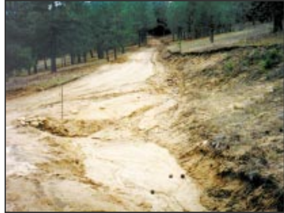
Poor drainage on granitic soils can deliver large amounts of sediment to streams.
