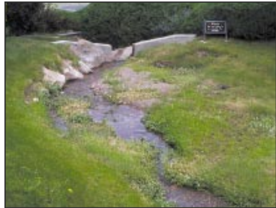
This small impoundment has filled with gravel and plants are taking hold.
