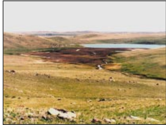
Hundreds of thousands of cubic yards of sediment have filled much of this reservoir.
