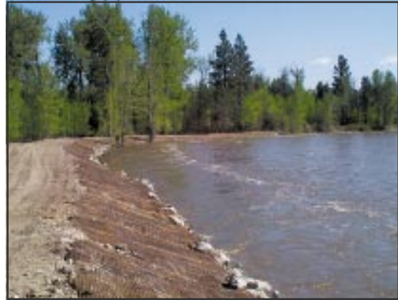
This levee was stabilized to protect downstream development from flooding, although the landowner with the levee did not particularly want to constrain the river.
