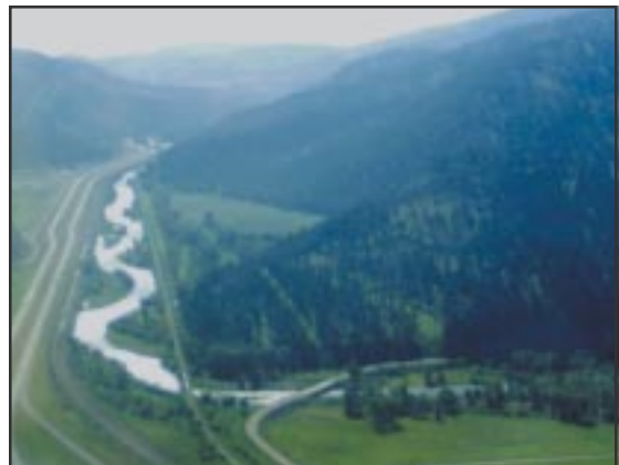
This river has maximized meander length given infrastructure constraints, but remains unstable over much of its length.
