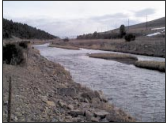
Channelized streams seek to re-establish equilibrium by forming meanders with scour and deposition. This stream is depositing sediment in an overwide channel, and is re-establishing a meandering, bankfull dimension channel.
