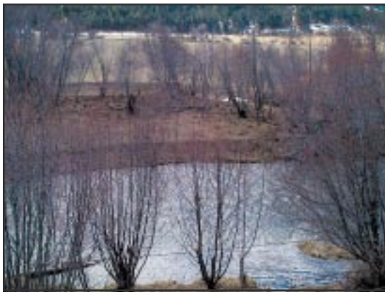
Comparing the elevation of the straightened channel and the old channel streambed (background) gives some indication of the degree of downcutting.
