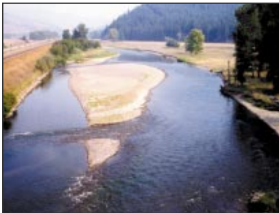
Rip-rap for bank protection is a common response to erosion on channelized rivers, but hard bank stabilization may prevent the river from re-establishing the missing channel length and stable meandering form.
